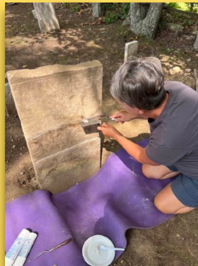
Lori Couture fills in a crack on the stone to prevent water infiltration.
