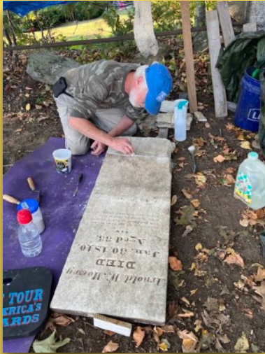
Mark Laprade does the infill on a repair to this tablet.
