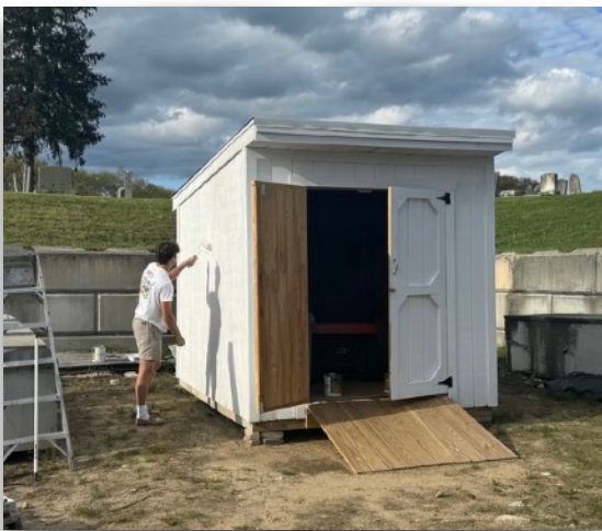
A volunteer has finished painting the cemetery shed.
